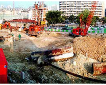
Construction of 134 housing units on the banks of the Ourcq canal for Bowfound Marignan in Paris 19th arrondissement Handover 2014
