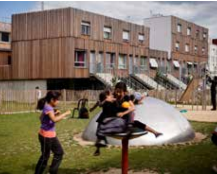
58 middle-class housing units at Valenton for Immobiliere 3F
